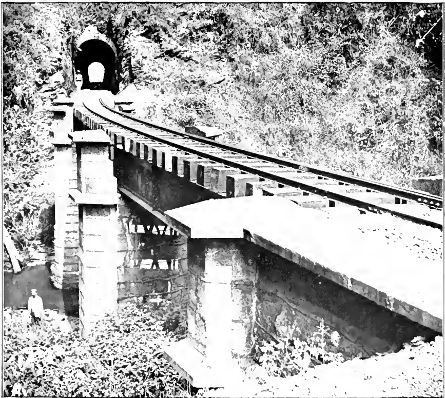
Central Railway of Brazil: Tunnelling through the Serra do Mar.
